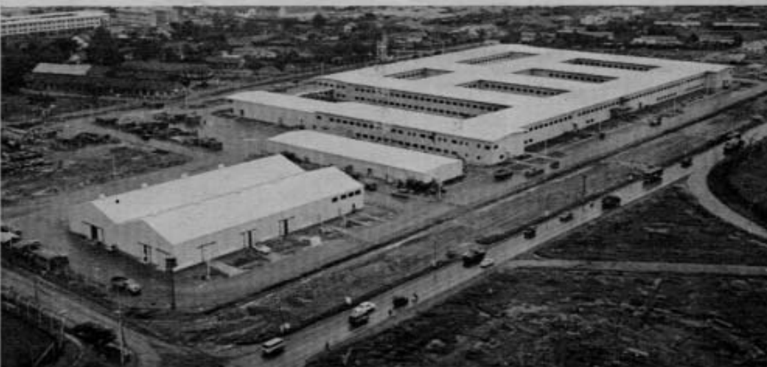
HEADQUARTERS SITE—The new USMACV headquarters building, completed in the latter part of the summer of last year, is located on a 23-acre site at Tan Son Nhut. In a sense, it is a small city as it has its own electric power plant, communications, water wells and sewage system. The two-story building contains the offices of COMUSMACV and his major staff officers. (USN PHOTO)
