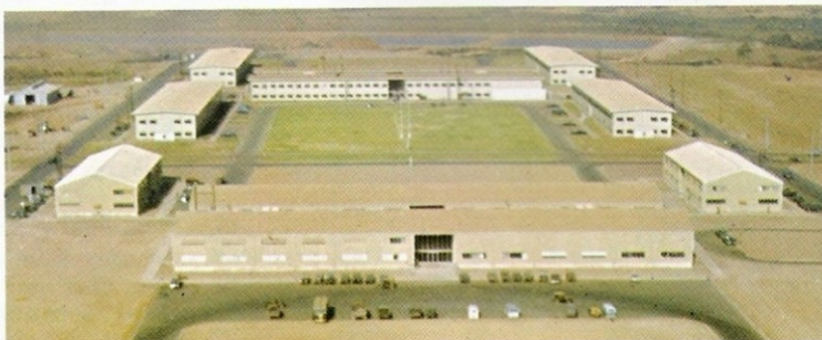
USARV and 1st Logistical Command headquarters buildings at Long Binh Post form a geometric pattern in what was once jungle. Photo by Sp4 James Lynch.
